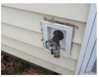
Recommendation: While no repairs are required, you may elect to update the outside faucet by installing a modern automatic draining, antifreeze type valve with a check valve to protect the public water supply from possible cross connection hazards. A competent and qualified plumber can provide you an estimate for this repair.
